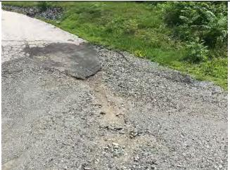
**Photo 1:** Sediment runoff directly into the Poultney **Photo 2:** Erosion in driveway at the toe of slope. River channel.
