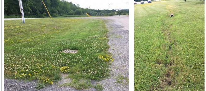
**Photo 1:** One of the three catch basins draining the school **Photo 2:** Minor erosion from outlet. driveway.
