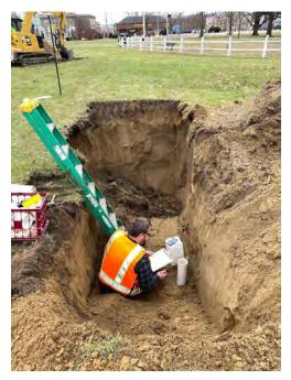
**Figure 3:** Project FHV-06 had the highest total score (31 out of 50) in the Unified Prioritization. The project is located on the north side of the Fair Haven. In fall of 2021 FEA and the Town performed test pits to verify soil suitability for a large underground infiltration practice.
