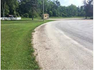
**Photo 1:** Sheet erosion in gravel portion of parking lot.
