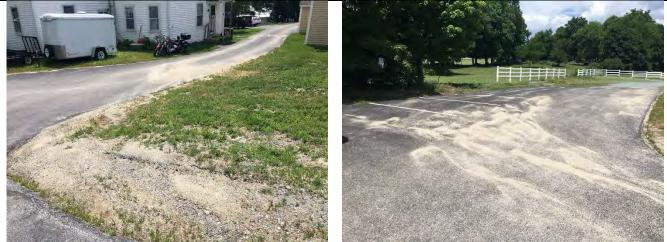
Photo 1: Corner of driveway being eroded and mobilizing sediment. Photo 2: Sediment from uphill deposited on paved driveway.
