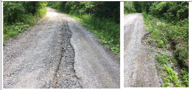
Photo 1: Gully erosion in center of the road from water flowing<br/>directly down ROW.Photo 2: Erosion from ditch overflowing<br/>into ROW.
