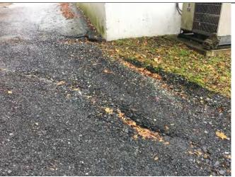
Photo 1: Stormwater flowing over gravel out of broken culvert Photo 2: Eroding gravel in driveway just uphill of low point
