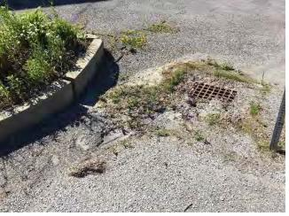
Photo 1: Sediment runoff along road edge.
