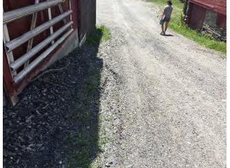
Photo 1: Deposited sediment from the coming from the<br/>corner of the parking lot.Photo 2: Small gully forming in steeper section of the<br/>parking lot.
